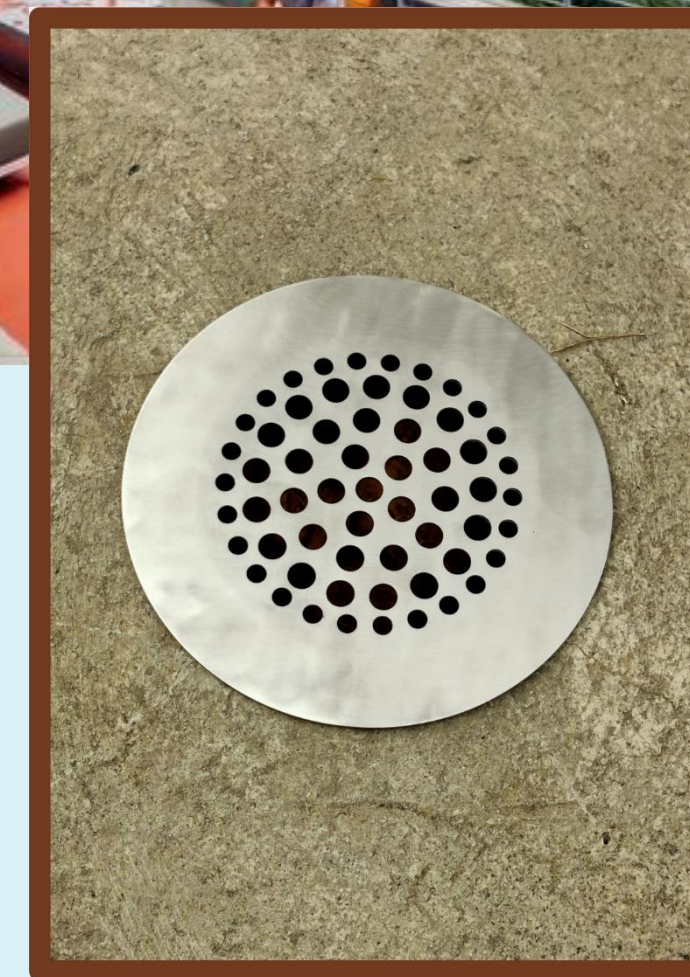
Cover Kunji Pit using a purpose-built stainless steel cover
